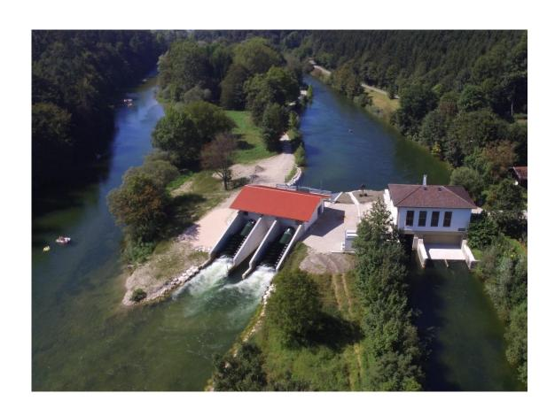
Water snail: power increase at existing hydropower; fish and eels can pass unharmed; plant on the Alz, north of Chiemsee in FFH area
